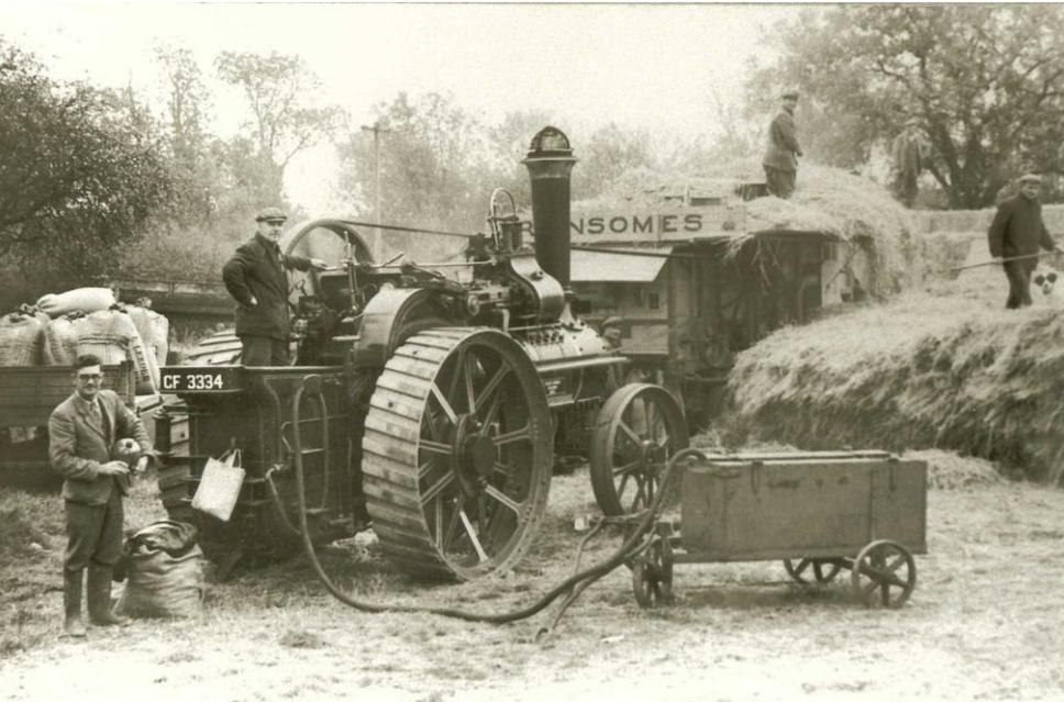
Steam engines were used on farms as early as the 1790s. These large engines were built in barns and used to drive threshing machines. These threshers separated grains from the chaff.
